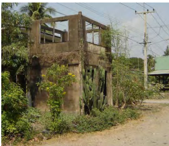
Figure 32 Two-storey railway substation
