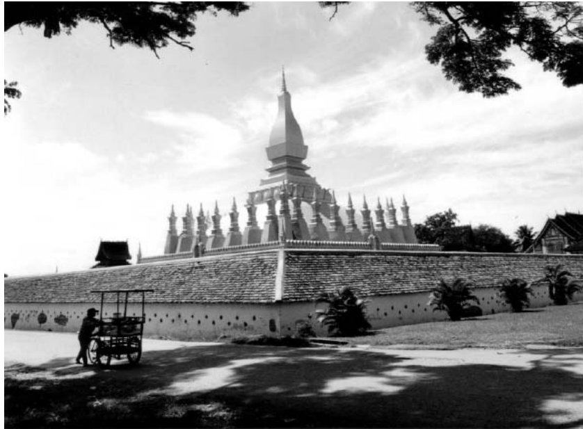
20. That Luang at present after the restoration by Louis Forbertain 244
