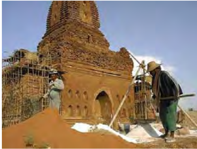
59. Restoration work at a pagoda in Pagan (Source: www.6foot6.com )
