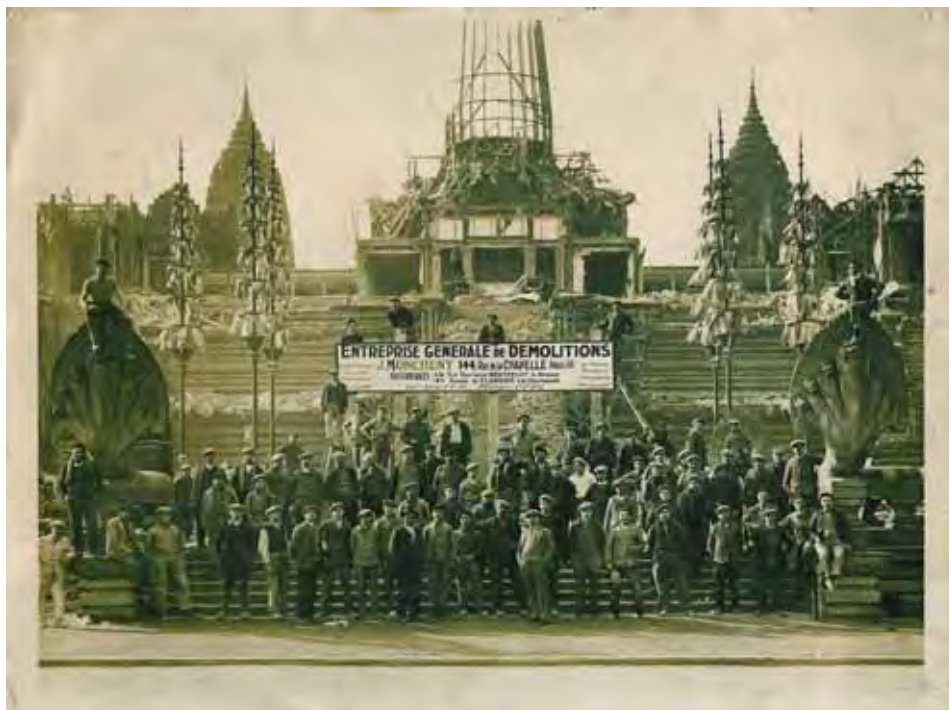
34. Angkor Wat Pavilion when being demolished (Source: unknown)
