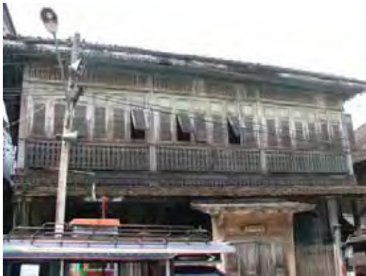
Figure 154: Boriboon House. ( Photograph: 28.03.2009 )
