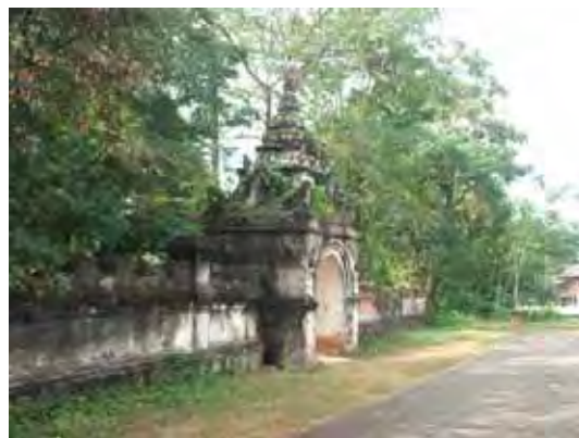
Figure 220: Condition of the second gatehouse with lichen and weeds growing on top.
