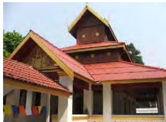
Figure 56: New monastery ( vihara ) with gable on double hip roof ( Jetawan type). ( Photograph: 17.11.2008 )
