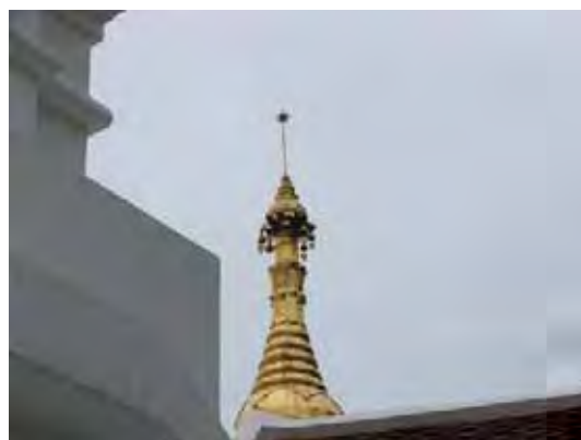
Figure 194: New metal ware on the pagoda. ( Photograph: 07.07.2009 )
