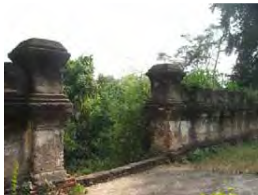
Figure 222: Condition of the wall.
