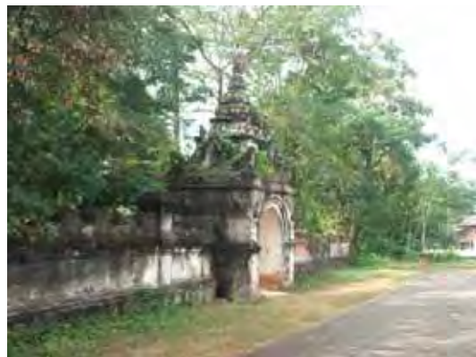
Figure 106: The porch entrance gate.
