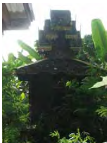
Figure 178: Condition of the toilet built with wood. (Photograph: 17.11.2008)
