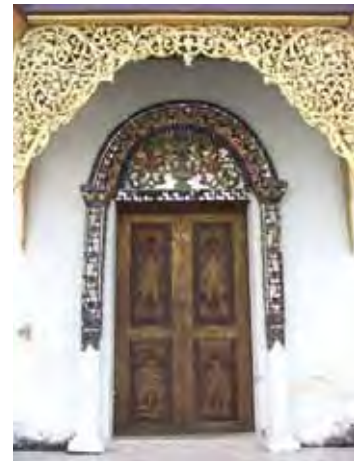
Figure 216: Complete decorated wood carving, colored glass mosaic and gild at the entrance of the small ordination hall. ( Photograph: 07.11.2008 )
