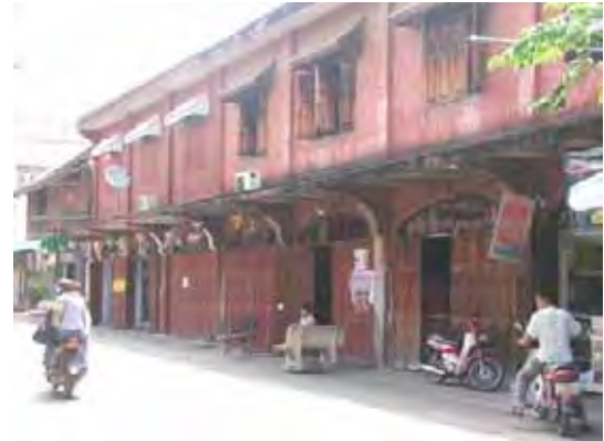
Figure 153: Tuek Dang or Red Building. ( Photograph: 16.02.2009 )
