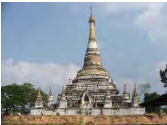
Figure 223: Condition of the easternmost pagoda. ( Photograph: 07.11.2008 )
