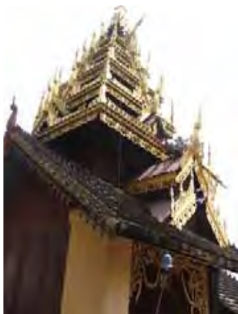
Figure 172: Condition of pythat roof. ( Photograph: 17.11.2008 )
