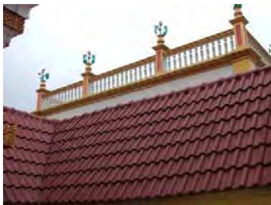
Figure 184: The upper part of European - style ordination hall with modern pantiled roof. ( Photograph: 19.02.2009 )
