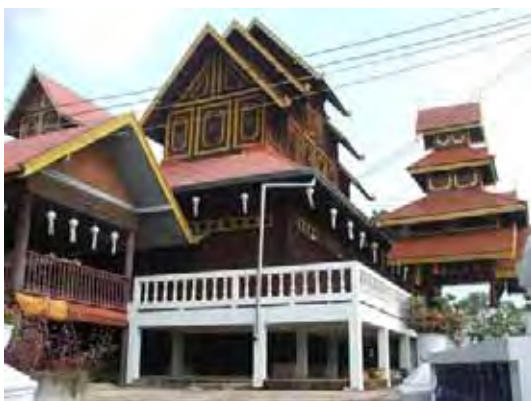
Figure 211: Condition of the monastery. (Photograph: 07.11.2008)
