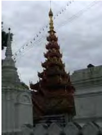
Figure 162: Zinc coated iron sheet with corrosion.
