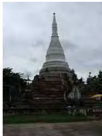
Figure 231: Condition of pagoda from the second survey.
