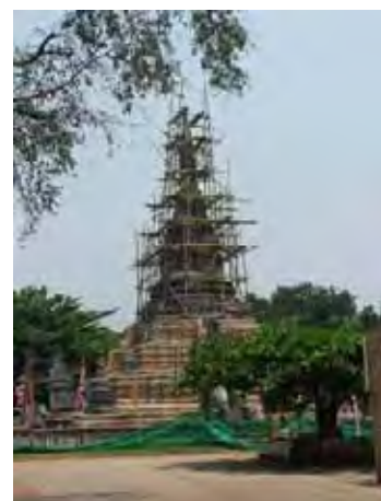
Figure 124: The pagoda in the process of renovation.
