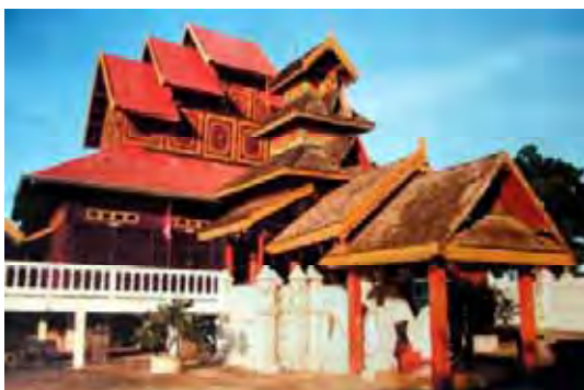
Figure 207: Condition of the monastery before restoration by Fine Arts Department. (Source: Fine Arts Department, 07.07.2009 )
