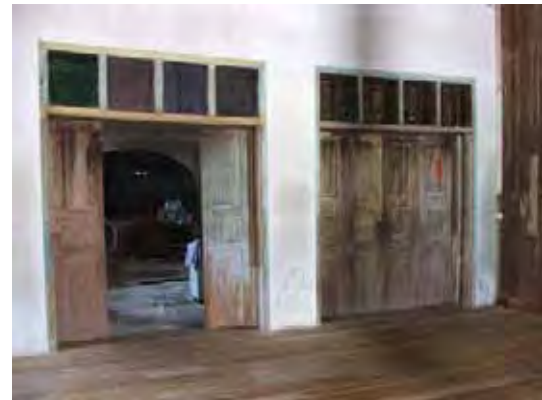
Figure 139: Vacant space on the first floor. ( Photograph: 16.02.2009 )
