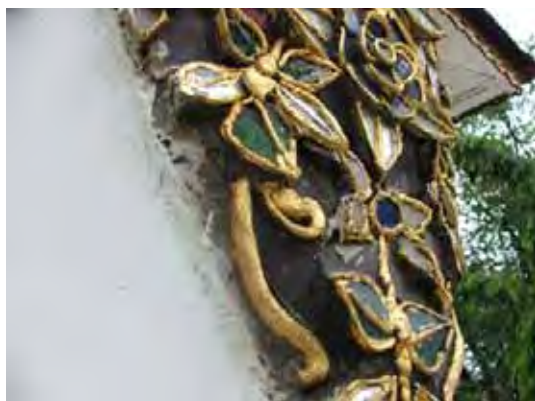
Figure 189: The use of epoxy bond to strengthen colored glass mosaic. ( Photograph: 07.07.2009 )
