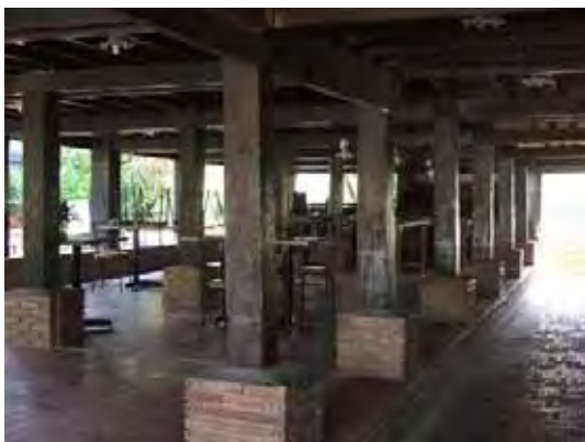
Figure 134: Numerous posts that are maintained by red brick.
