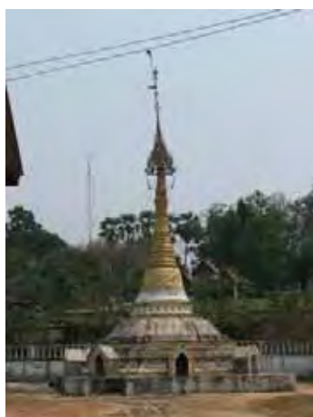
Figure 229: Condition of pagoda. ( Photograph: 29.03.2009 )
