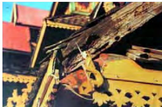
Figure 210: Decayed wood before restoration by Fine Arts Department. (Source: Fine Arts Department, 07.07.2009)
