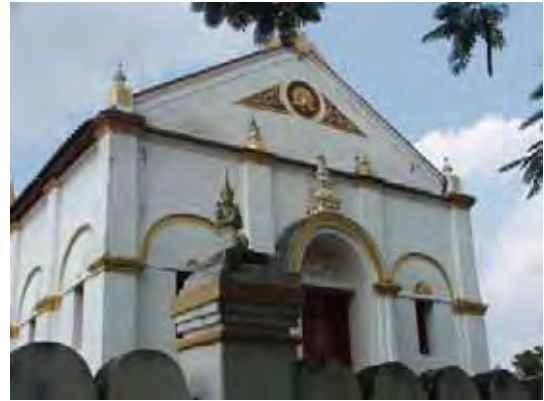
Figure 214: Condition of the vihara. ( Photograph: 07.11.2008 )
