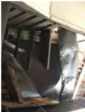
Figure 132: Iron sheet under the roof of Ban Sao Nak.
