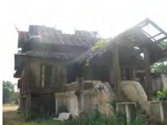
Figure 224: The northwest view of greatly ruined monastery. ( Photograph: 07.11.2008 )
