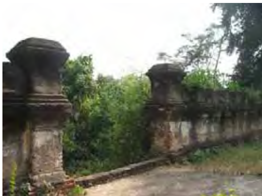
Figure 105: The boundary wall.
