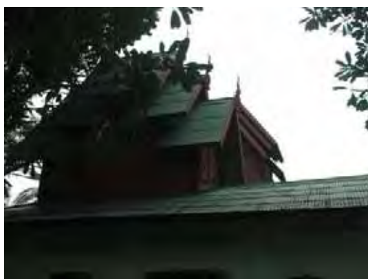
Figure 187: Condition of the roof of monastery. ( Photograph: 29.03.2009 )
