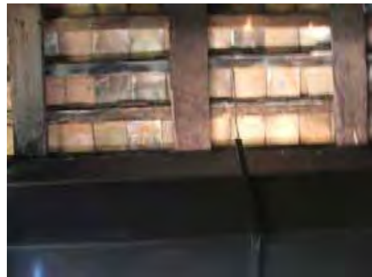
Figure 131: Terracotta tiles with a perlin hook.
