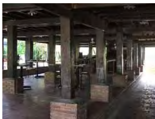
Figure 235: Addition of concrete plinths.
