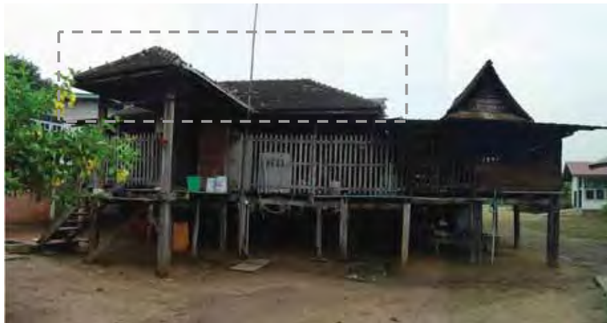
Figure 59 Example of a hip roof in Pakkran village
