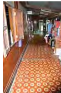
7.4 Right side corridor
