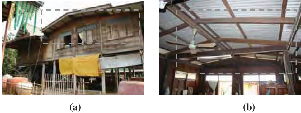
Figure 58 Structure of a bungalow roof of the sample in Pakkran village
