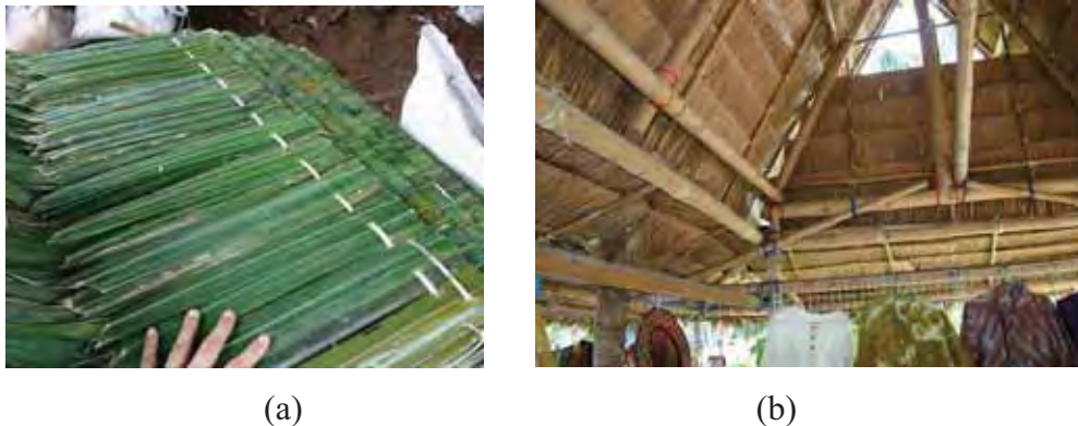
Figure 79 Thatched materials in the traditional group: (a) palm leaf and (b) grass (Source: Temporary shelters in the surveyed locations)
