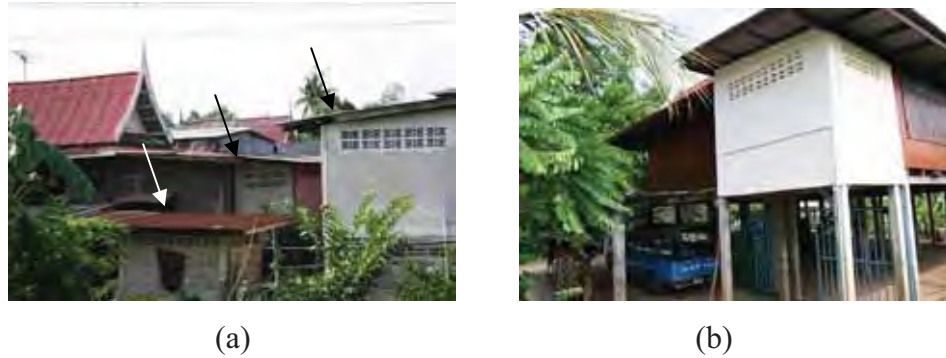
Figure 69 External and internal bathrooms
