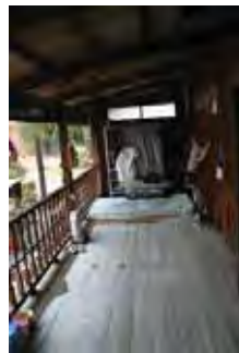
7.3 New front terrace
