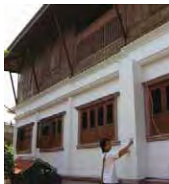
Figure 89 Contemporary columns clad with plaster, bricks, and plaster ornaments
