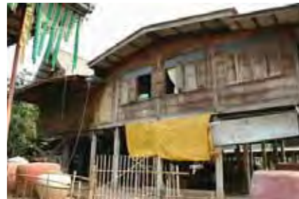
8.2 Left side facade
