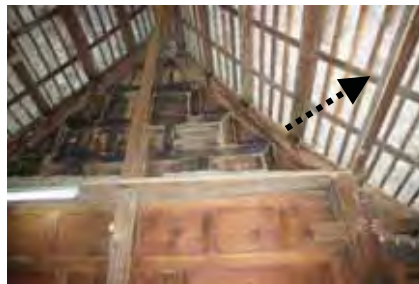
Figure 48 Curved rafters, purlins and battens
