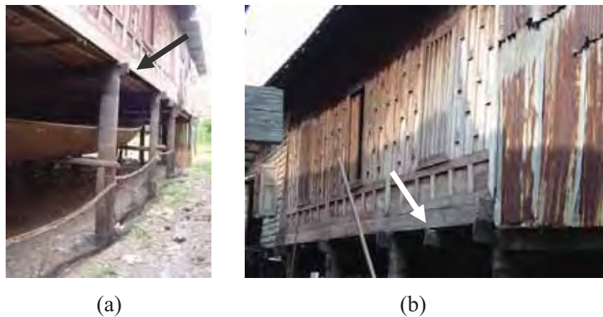
Figure 91 Upper level beam: (a) Traditional beam and mortised column, (b) Supporting beam between the main traditional beams
