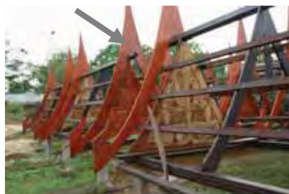
Figure 82 Bargeboards of the traditional roof structure
