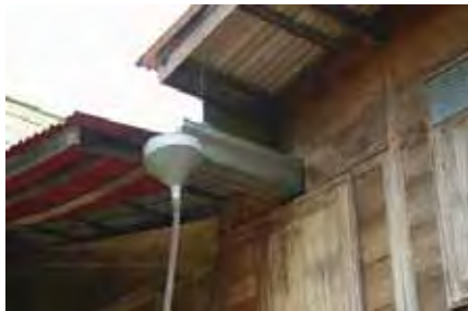
8.1 Wall, roof, gutter and down spout
