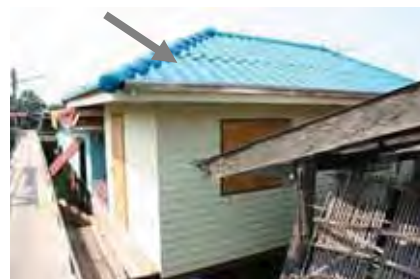
Figure 83 Hipped roof of a vernacular house in Ladchado village
