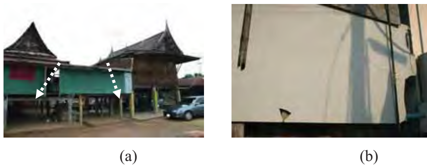
Figure 54 Change of wall panels at sample in Pakkran
