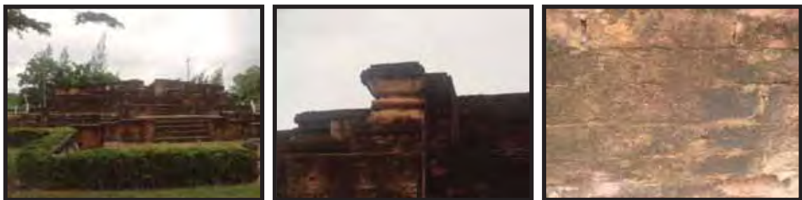
a. Chedi of Wat Vieng (left and middle) b. A technique of brickwork without grouting of Srivijayan art (right)
