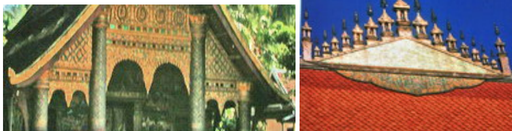
Figure 16: Pediment decoration with Luang Peung (honeycomb) in general Lao temples in Lao PDR (left). The decoration on the top of the roof, dok chor fah (right).
