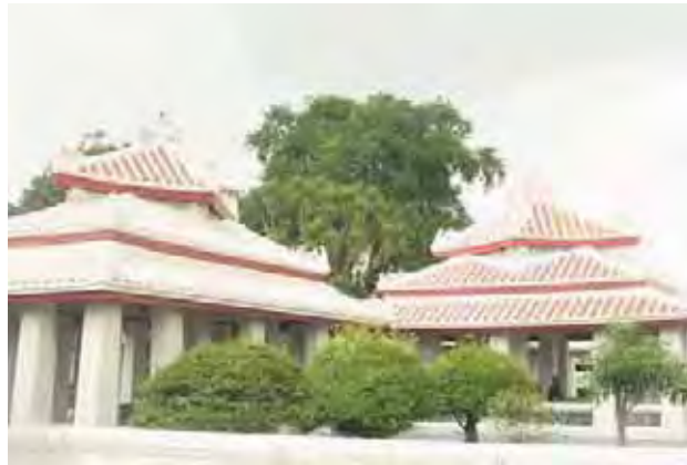
Figure75 : Riverside pavilions Photograph by: Kanjanaphorn Polprateep : June, 2008
