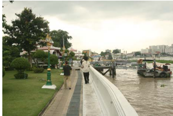
Figure 109: The dam for preventing flooding at Wat Arun Photograph by: Kanjanaphorn Polprateep : May, 2008.
