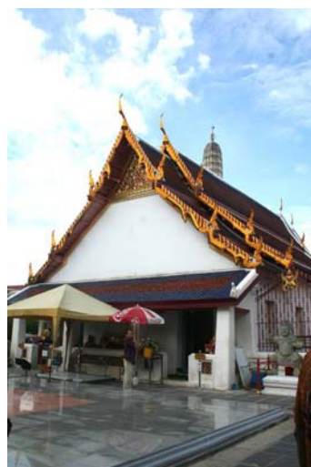
Figure 97: The pavement in front of Viharn-noi or the small chapel after adaptation
