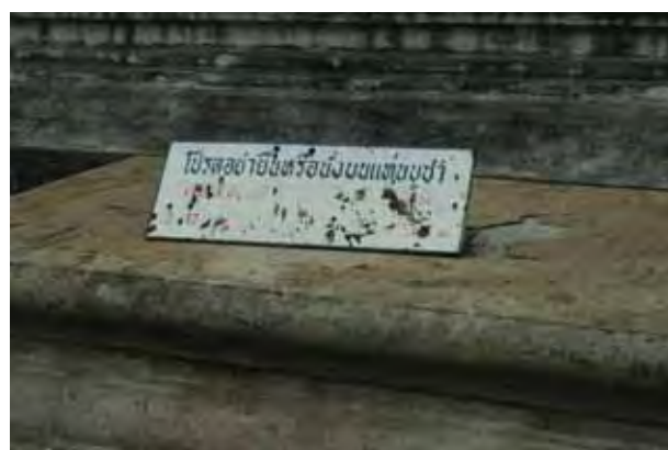
Figure 129: Decayed sign which English cannot readable on site for telling visitors not to stand or sit on the sacrificial stone
