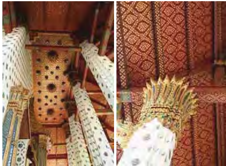
Figure59: The outer ceiling (left)
