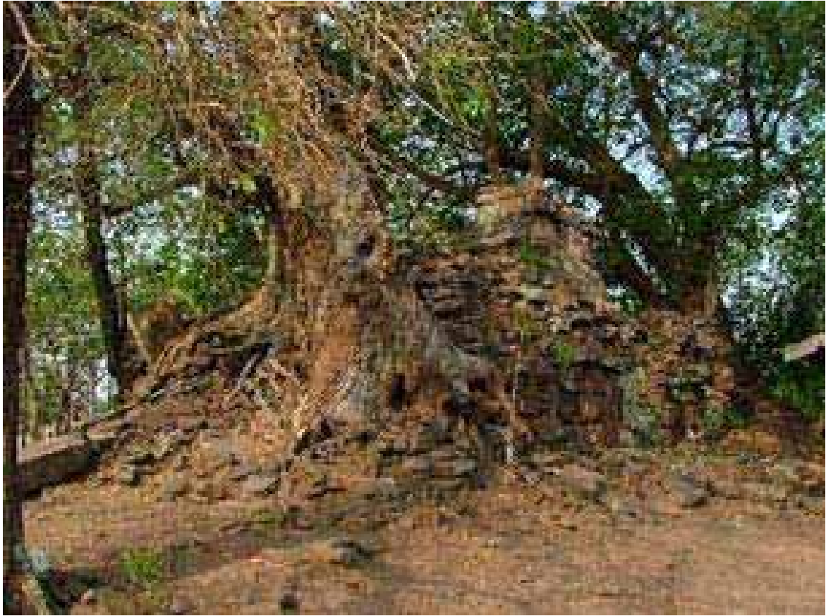
Fig. 10 Ruins of Dharmasala No. 17 on the Dharmasala Route or Royal Route from Angkor to Phimai. Prasat Ku Sila Khan, Khorat Province, Northeastern Thailand. Photo: Asger Mollerup
