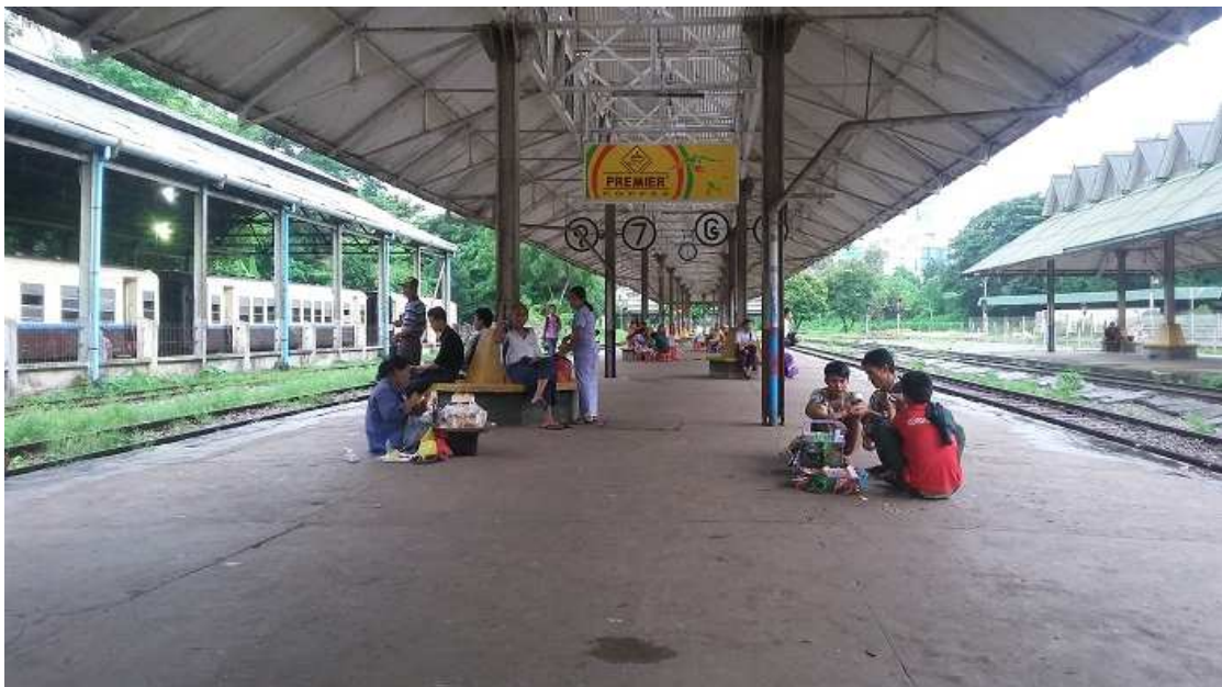
Figure 3.2 Yangon central train station (Research setting 2)
