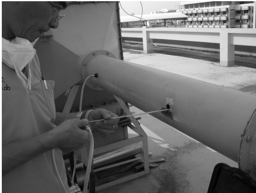
D6 Measuring air velocity approaching to the filter by probe
