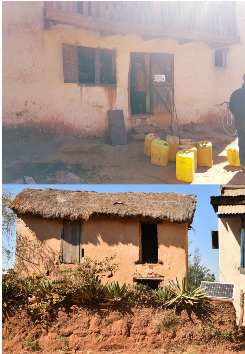
Figure 11.4: Fighting the absence of Water and Electricity supply Source: Mbola, 2017
