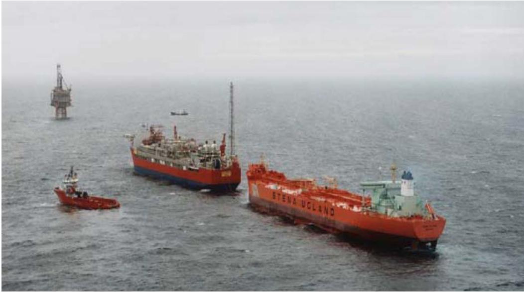
Figure 2.1 Store liquefied natural gas which transferred from the central processing platform (CPP) [9]
