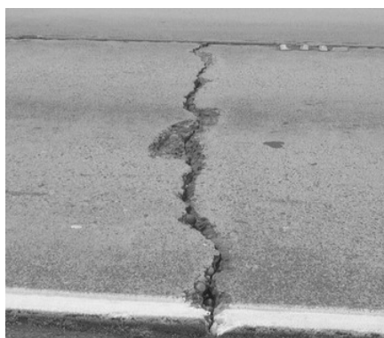
Transverse Crack
