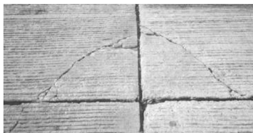
Corner Crack
