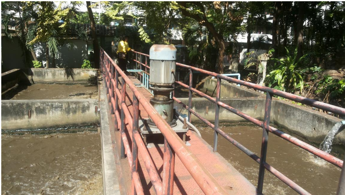
Fig. A.19 The aerator tank of hospital C.
