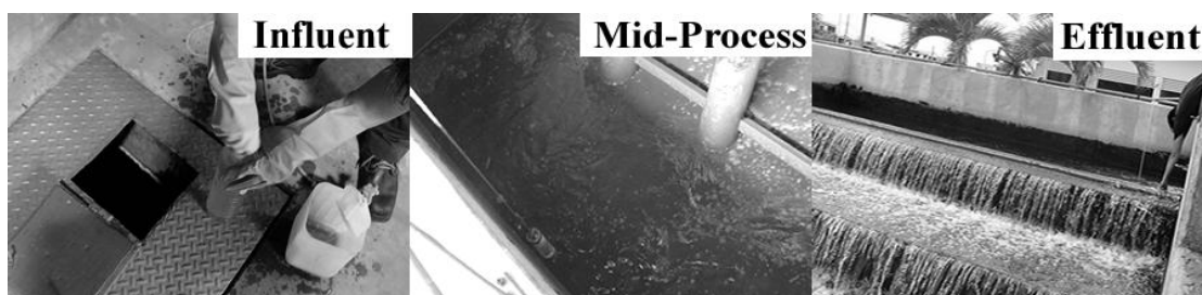
Fig 3.5 Sampling Points of ChongNon Si WWTP (CN)
