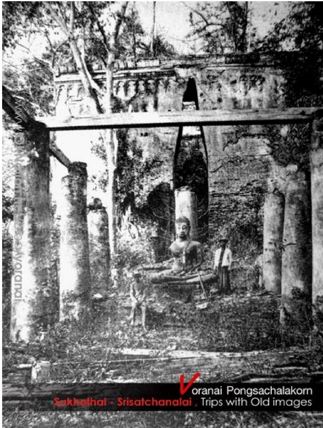
Fig. 53 Vihàra of Wat Si Chum which remained the wooden beams on top of mortar pillars and the Acana Buddha image's pavilion in the background.
