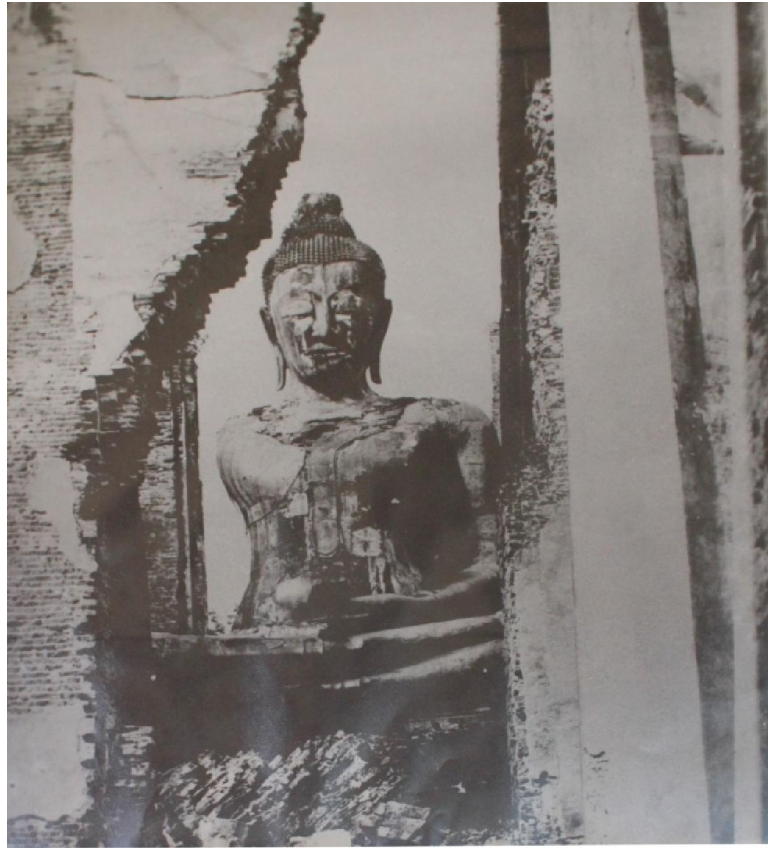
Fig. 62 The photo of Phra Mongkhon Bophit without the right arm and topknot of Buddha image deteriorate before restoration process can be seen at the wall inside Vihàra Phra Mongkhon Bophit.
