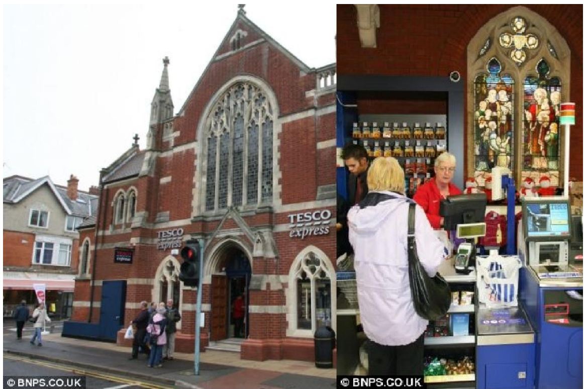
Fig. 47 The current exterior and interior of Tesco Express which is the former Methodist Church in Westbourne.
