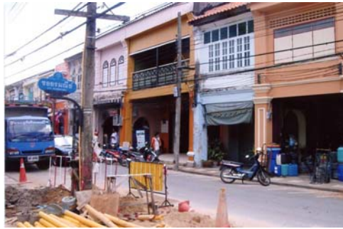
Figure 184: Bury power cables on Thalang Road underconstruction Photograph: Author, 2009
