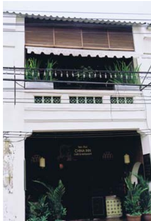
Figure 45: Hub Long Huat Building Photograph: Author, 2009
