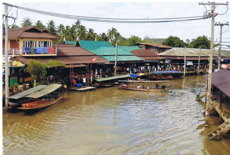
Figure 143: Row – Houses along the canal in Amphawa
