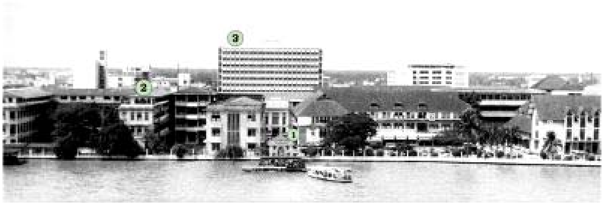
Figure 46: Development of Siriraj Hospital, 1971
