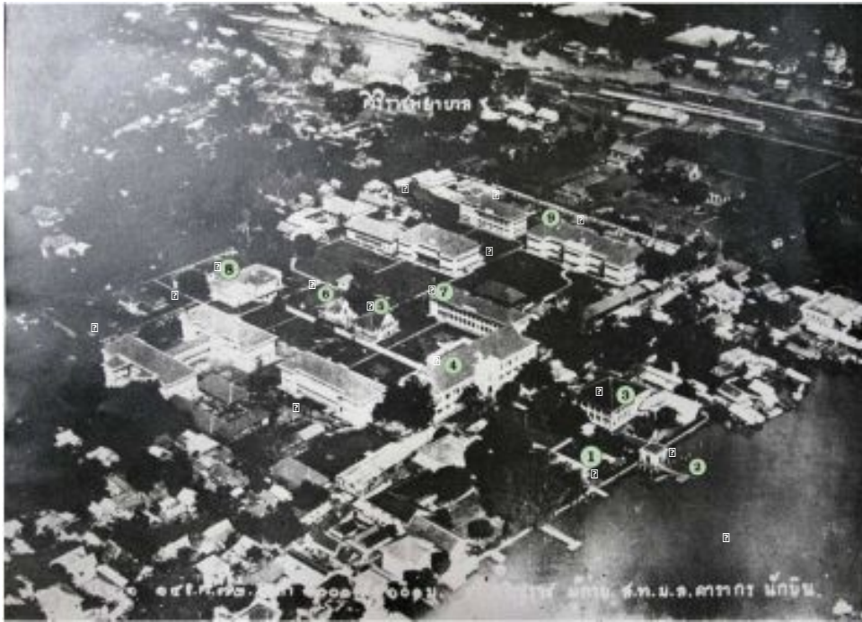
Figure 32: Development of Siriraj Hospital, 1929
