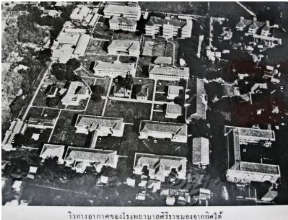
Figure 34: Development of Siriraj Hospital, 1935
