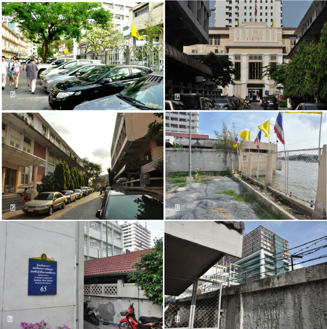
Figure 82: Fences and walls within Siriraj Hospital
