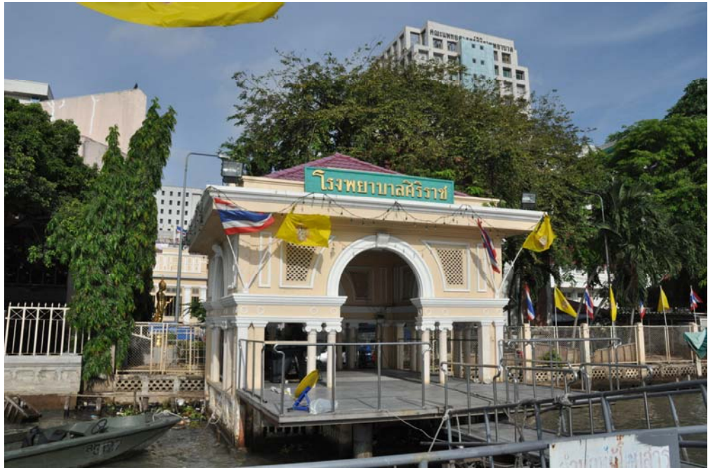
Figure 65: Siriraj Pier, built in 1923.
