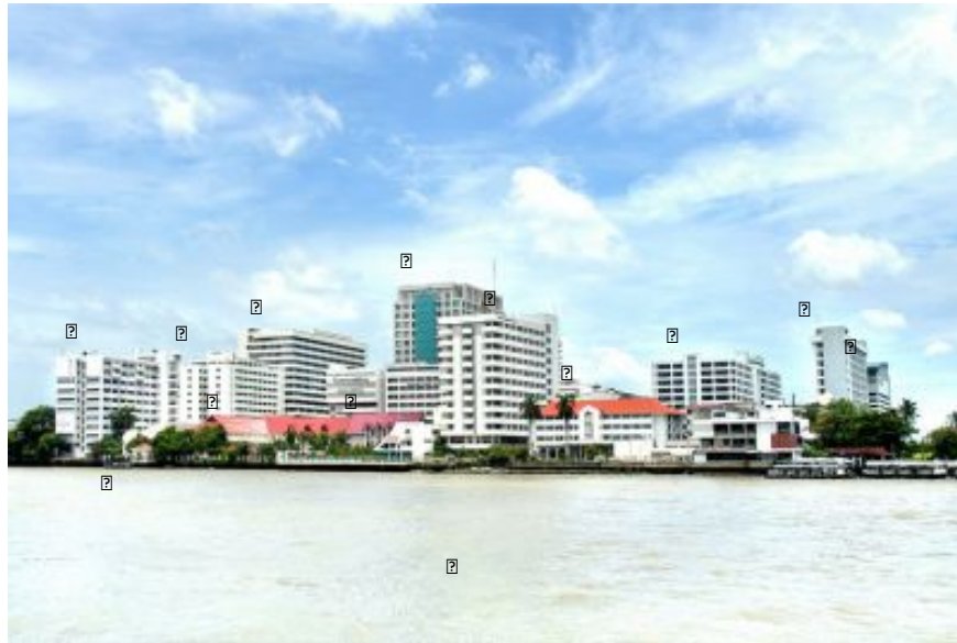
Figure 54: Development of Siriraj Hospital, 2005
