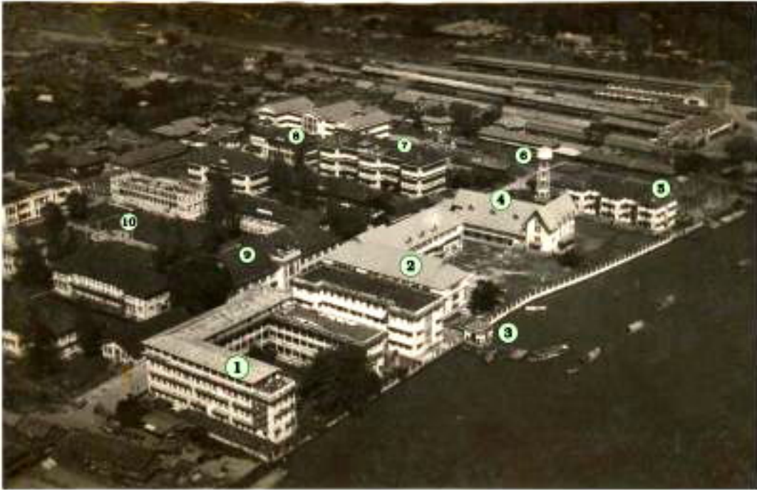
Figure 41: Development of Siriraj Hospital, 1957
