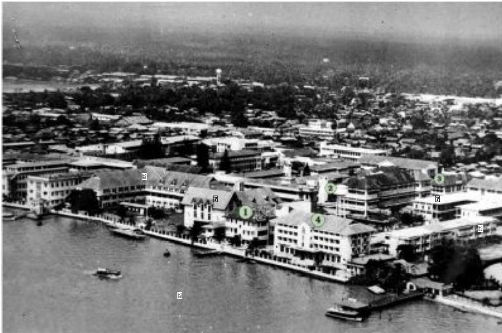
Figure 44: Development of Siriraj Hospital, 1964
