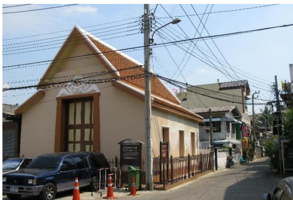
Figure 100 The original Conception Church built since King Narai period in Dutch architectural style. Photograph by Phungwong, N. July 16, 2010.
