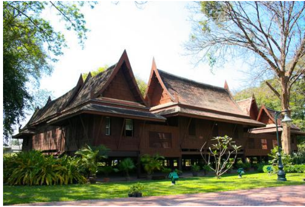
Figure 153 Photograph of a traditional Thai house. Ruern Tab Kwan owned by Silpakorn University, Nakorn Pathom campus. The traditional Thai house was built with an integration of pavilions of various functions with an open ground floor. Moreover, it used wood columns and beams to carry the load. The roof gable is even sharper than 60 degrees. Photograph by Phungwong, N. on April 13, 2010.
