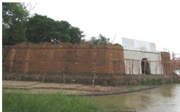
Figure 76 Pomphet (Diamond Fort). This fort was made from latelite and large bricks with a very strong foundation. This fort was the most important and largest among forts in Ayutthaya. In the beginning of the city, the city wall and fort was made from clay and wooden columns. It was reconstructed in bricks and stones during the reign of King Mahachakkaphat (1548-1568). He also built a large fort at the junction of the Parsak and Lopburi Rivers, Marhachai Fort to protect against enemies from the north. Photograph by Phungwong, N. on Jun 12, 2010.
