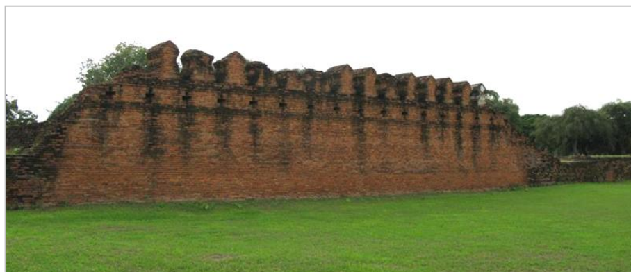
Figure 28 The remains of the Ayutthaya wall are seven meters high and ten meters in depth (foundation) in original formation. It is the last remain part of old city wall. Photograph by Phungwong, N. on May 1, 2009.
