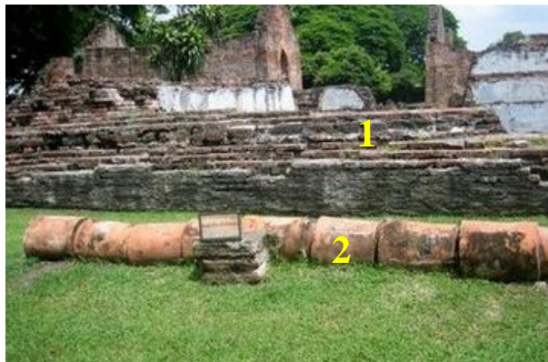
Figure 189 A water tank (1) and pottery water pipe (2) built in the King Narai Palace, Lopburi. The water pipe was constructed by a French engineer. They introduced waterworks between 1682-1684 starting at Lopburi and around 1685-1686 at the Ayutthaya palaces. Photograph by Phungwong, N. in February 2011.
