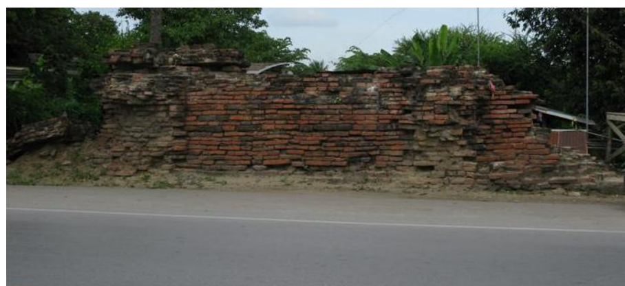
Figure 29 Above and below photograph shows the present day road around Ayutthaya Island built over the ancient Ayutthaya city wall. It was built in 1955 by a command of General Plak Piboonsongkram, Prime Minister of Thailand. Photograph by Phungwong, N. on May 1, 2009.
