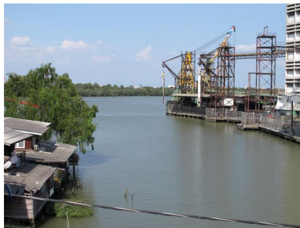
Figure 123 The mouth of Bang Pra Kod canal which had a large community in the late Ayutthaya period. Today on the right side is Mitpol's Sugar warehouses and left is local people houses. Photograph by Phungwong, N. on October 21, 2011.
