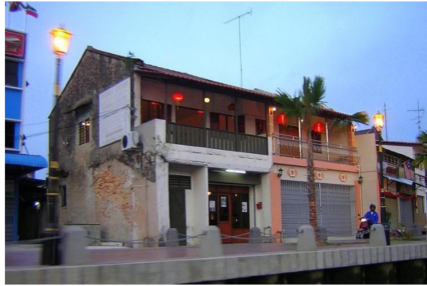
Figure 156 There are houses and shop houses in Malacca influenced by the Dutch farmhouse style. There are a lot of shop houses today in Thailand similarly influenced by the Dutch architectural style. Photograph by Phungwong, N. in December 2009.
