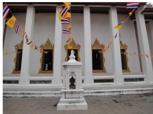
Figure 98 The exterior wall of the ordination hall (Bhakhakanok 15/7/2011)
