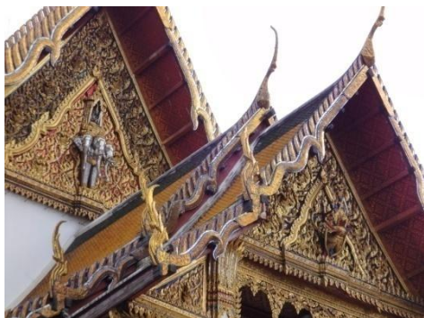
Figure 54 The pediments of the image hall (Bhakhakanok 6/6/2010)
