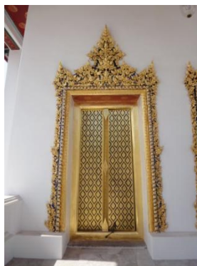
Figure 126 and 127 The exterior decorations (Bhakhakanok 25/12/2011)
