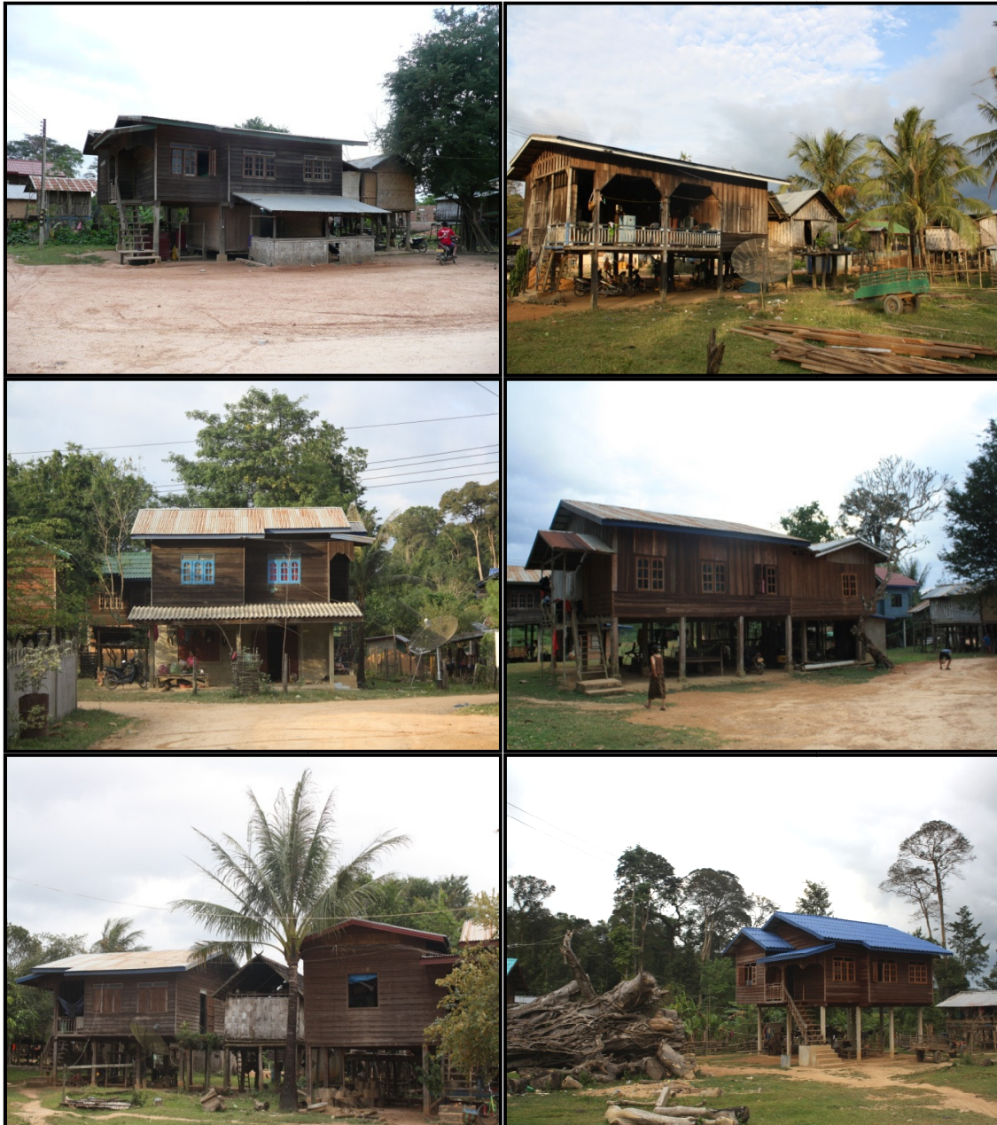
Figure 38: Half Renovated Phu Tai Houses (Photograph 28.11.2011)
