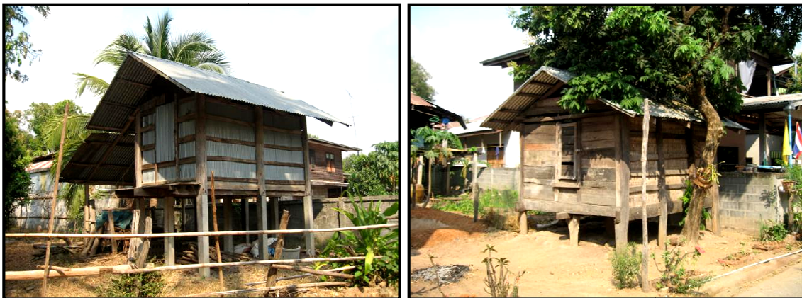
Figure 70: The Barn separated from the house (Left) The High Space Barn (Right) The Low Space Barn (Photograph: 14.07.2011)
