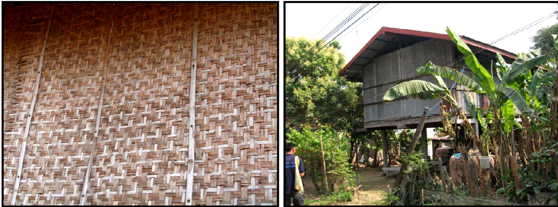
Figure 69: Original Style Phuthai Houses (a) – (b) The Two-Floor Bamboo House (c) The Bamboo Panel Wall (d) The Temporary Fence (Photograph: 28.02.2009)
