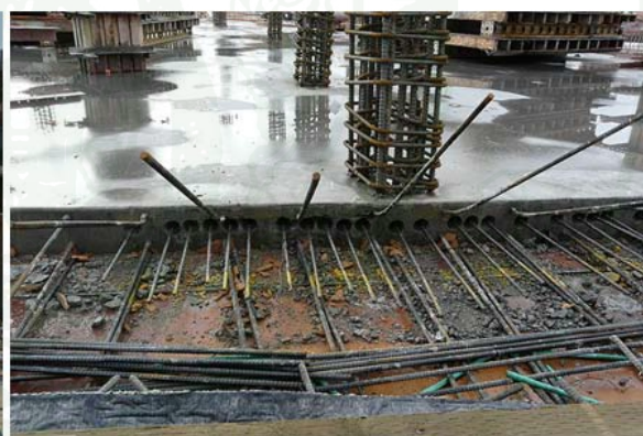
(4.3) Casting of concrete and curing 2
