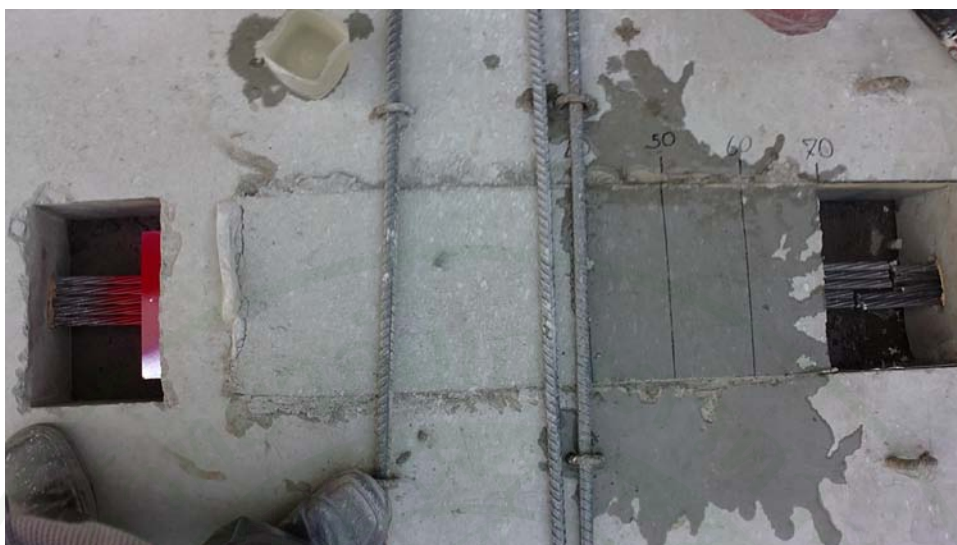
(a) Cutting all strands at the right end anchorage. Anchorage force transfer to the concrete in bonded length box
