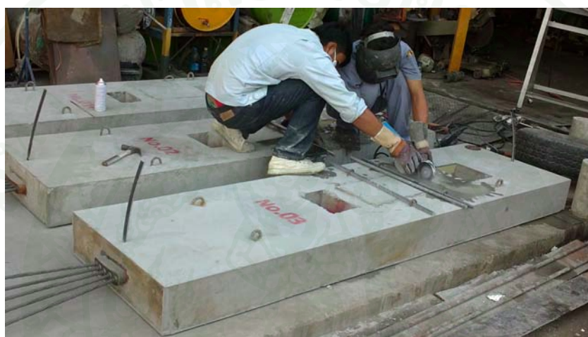
(a ) Cutting of the concrete 10 cm, step by step, to decrease the bonded length.
