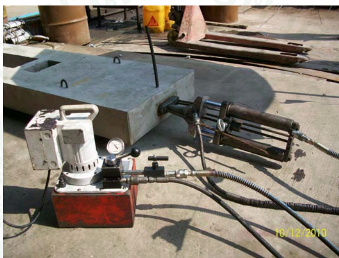
(a) Stressing of 15.0 ton/strand by jacking machine.
