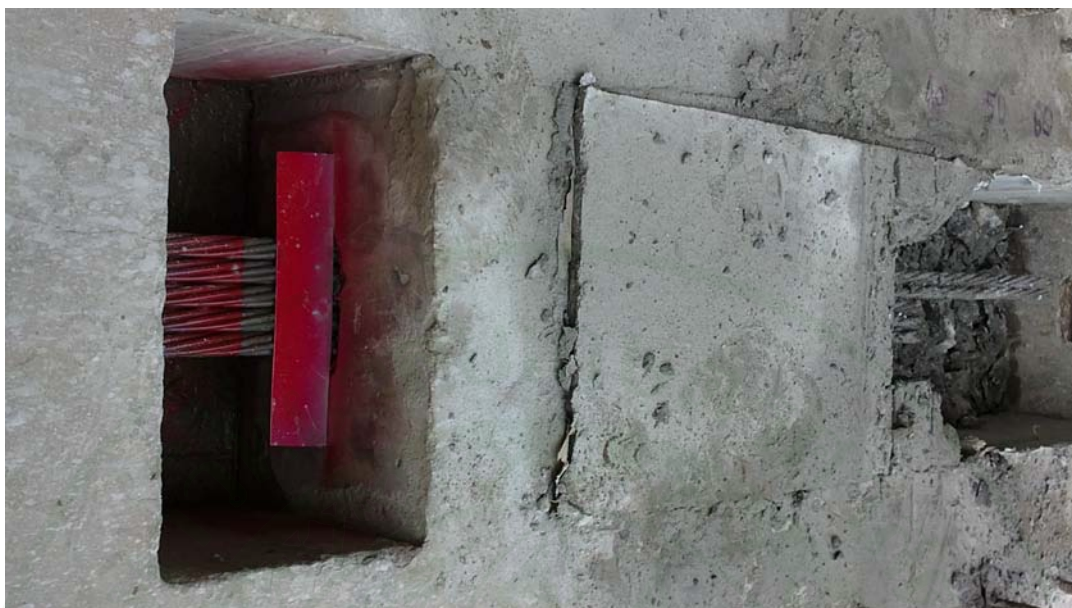
(a) Shows a failure of concrete at bonded length box after test.
