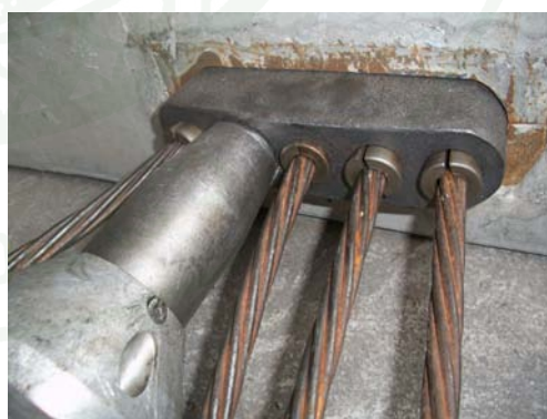
(c) During Jacking
