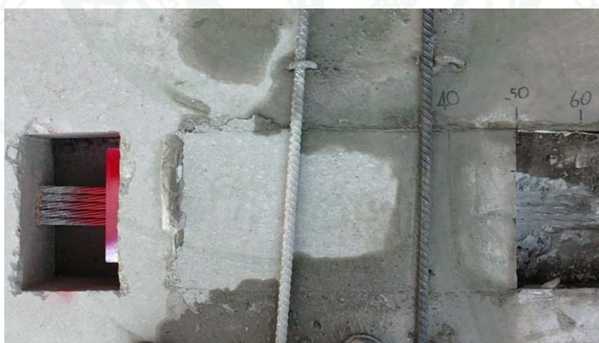
(b ) Each step of 10 cm cutting, step by step, checking slip as in step 3.7
