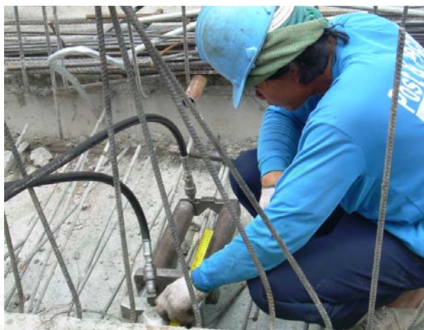
(4.4) Stressing tendon, tensioning of tendons and fixing of anchorage 2
