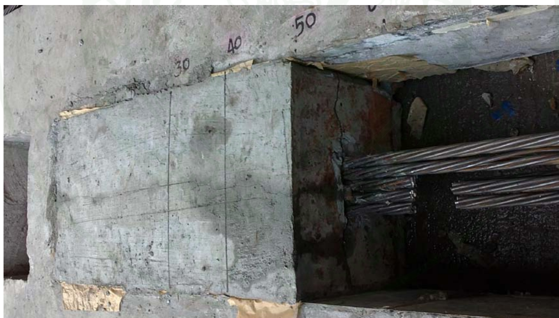
(b) Shows a failure of concrete in bonded length box after test.
