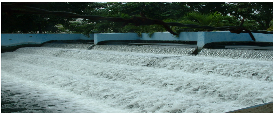
Figure 4.1.2 The cascade outfall of treated effluent discharged to Chao Praya River.
