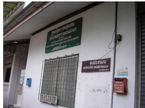
Picture 20: Community health center
