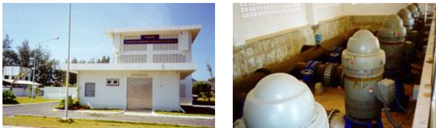
Figure 4-4 The building of water pump machines of the seawater irrigation system for marine shrimp farming in Kung Krabaen Bay
