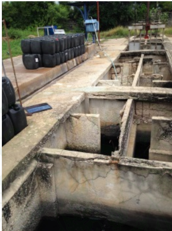
Appendix Figure D1 pH adjustment unit by adding \text{H}_2\text{SO}_4
