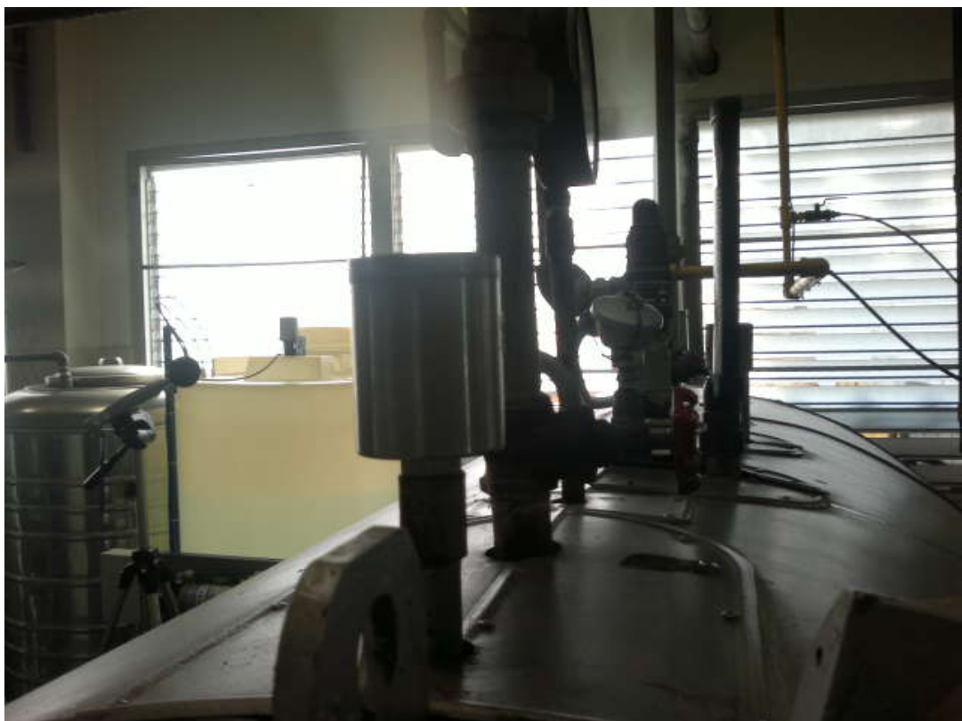
Figure A-7 Install silencer on retort.
