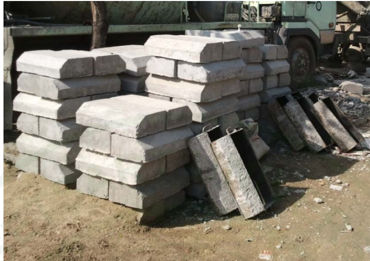
Figure 19 Reused leftover concrete in road construction purpose
