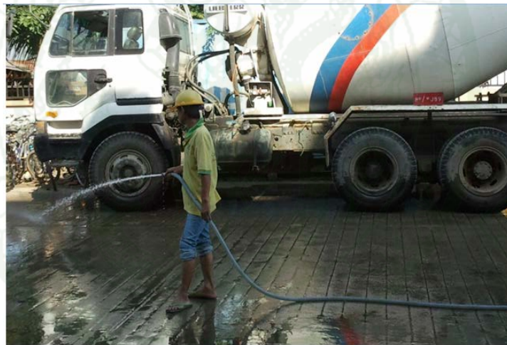
Figure 12 Concrete paving in CBP
