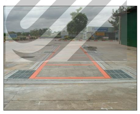
Figure 2.2 Foundation Semi-pit type
