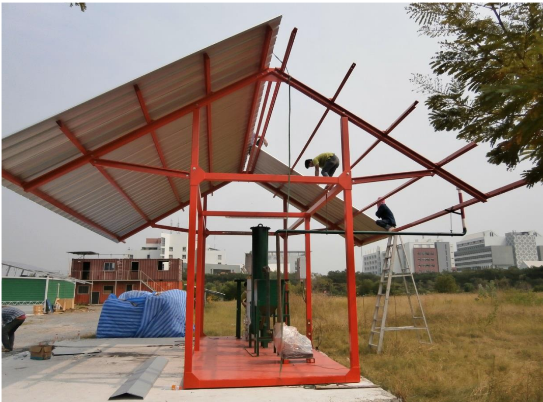
Figure 4.11 The Roof and Electricity Installation
