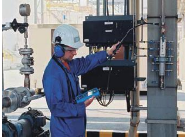
Figure 4.1 Monitoring air leaks by using Ultra Sonic Leak Detectors
