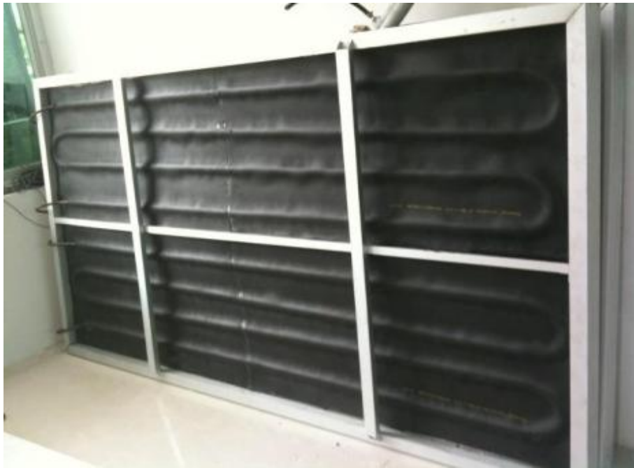
Figure A.1 A photograph of chilled water tubes behind the radiant panel.
