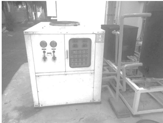
Figure 3.8 Heat pump of the building cooling system.
