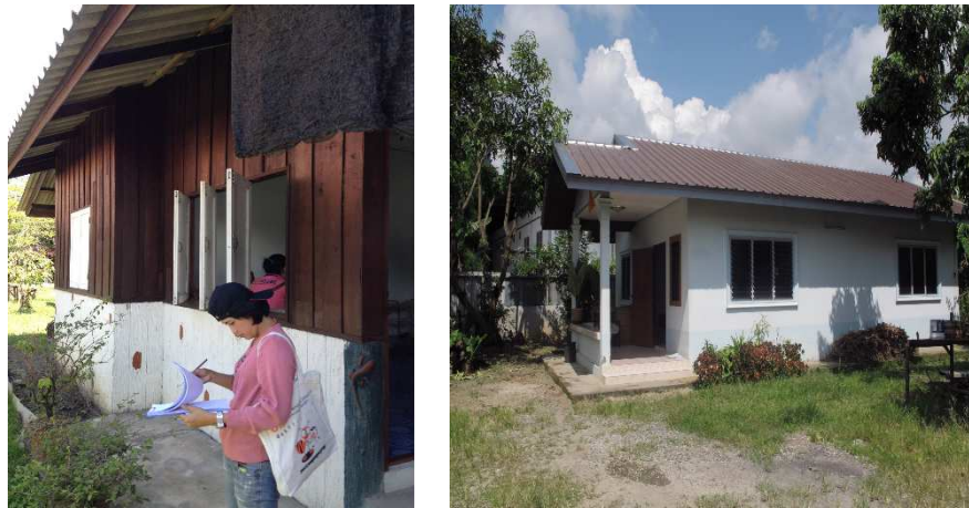
Figure 5.2. A house constructed with wood and concrete block and cement (a) and a house constructed with concrete block and cement (b).
