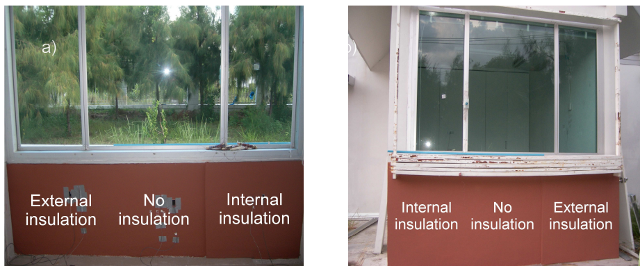
Figure 4.2 Photographs of interior and exterior configurations of the southern windowed wall, a) Interior, b) Exterior
