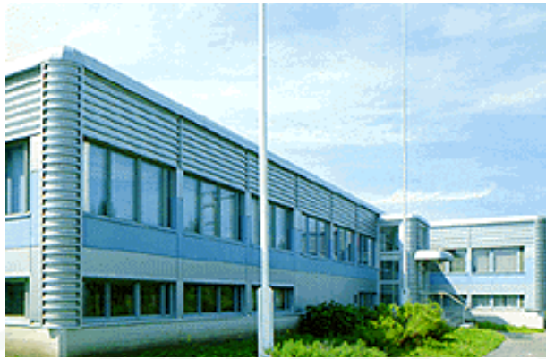
Figure 3 A facade made with profiled steel sheeting
