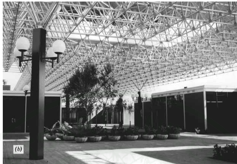
Figure 4 Cold-formed steel sections used in space frames
