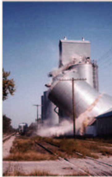
Figure 1.3: Collapse of a silo due to a poor design [22]
