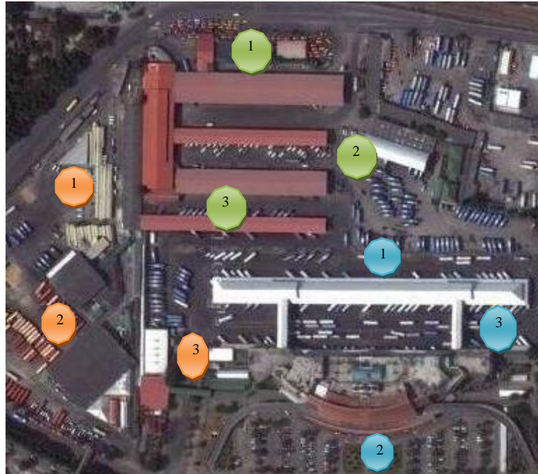
Figure 4.5 Location of Equipment Installation at Mho Chit II Bus Terminal
