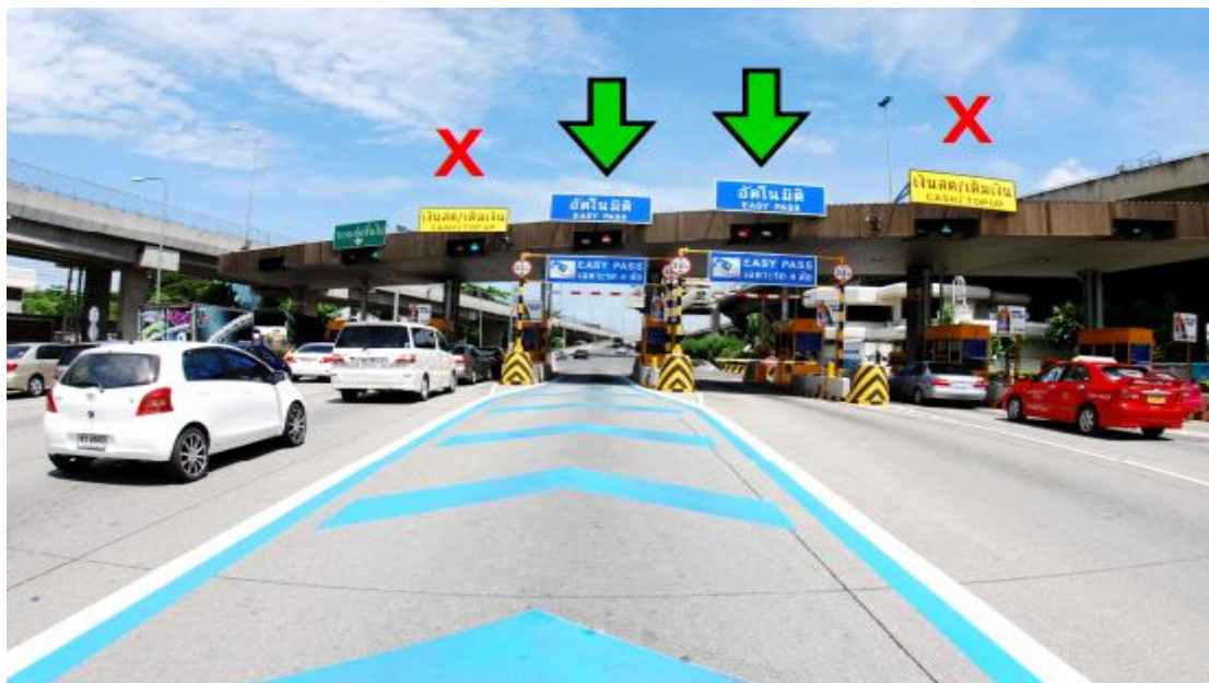
Figure 2.8 ETC in Thailand
