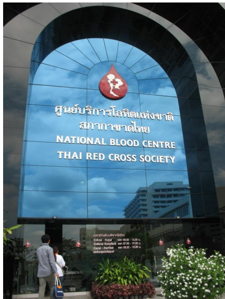
Figure 4.1 The head quarter building
