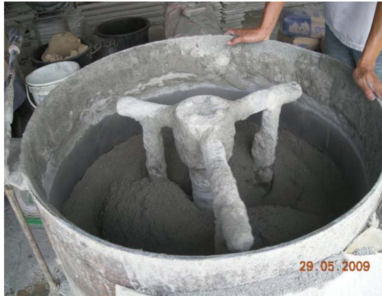
Figure 3.3 Mixture mixed in concrete mixer
