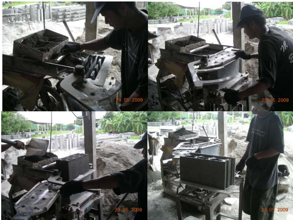
Figure 3.5 Making the hollow concrete block
