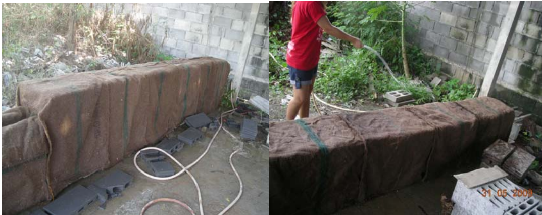
Figure 3.7 Curing the hollow concrete block
