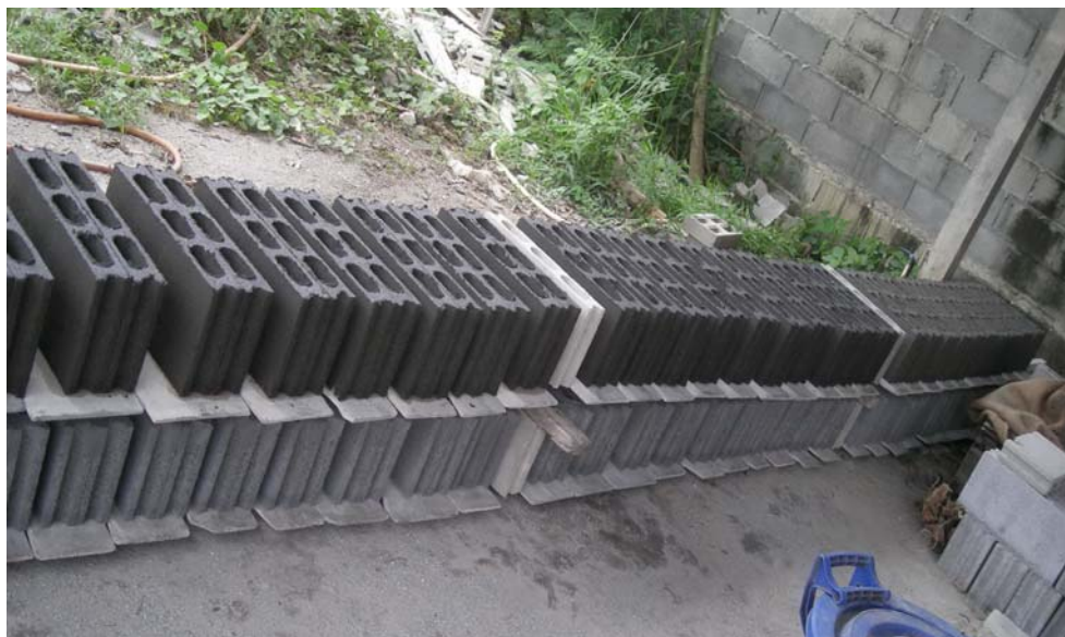
Figure 3.6 Dried the hollow concrete block
