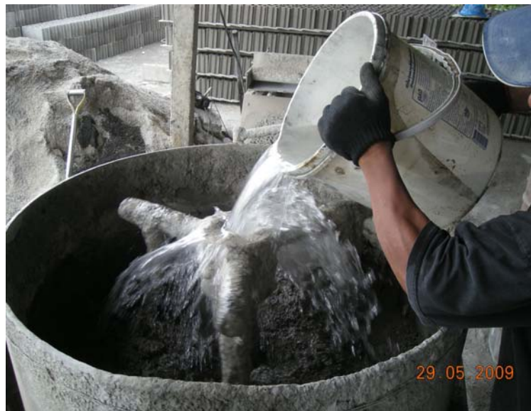
Figure 3.4 Water added into the concrete mixer
