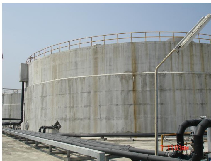
Figure 3.1 Anaerobic fixed film Reactor (AFFR) for biogas production system in tapioca starch manufacturing
