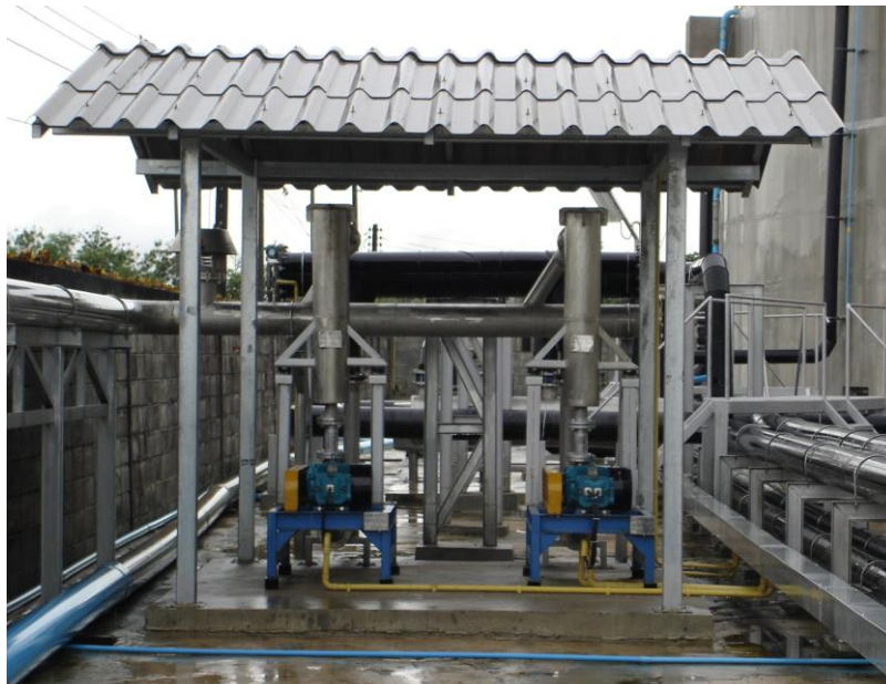
Figure D.1 Roots blower
