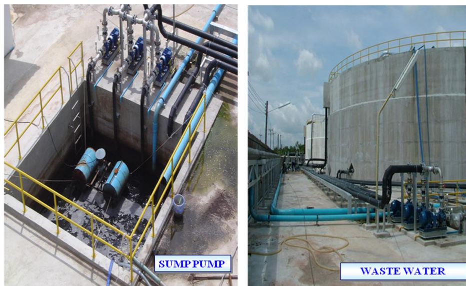
Figure B.1 wastewater pump and piping
