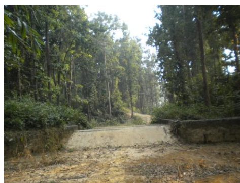
Upstream conservation/Masonry check dam and forest protection
