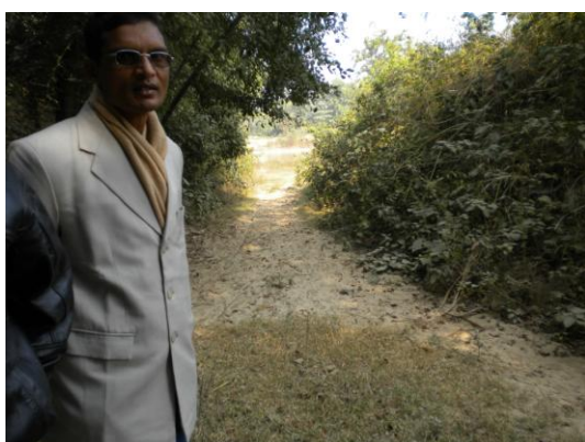
Water conveyance/Earthen canal
