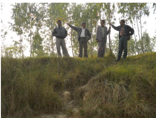
Downstream gully bank stabilization
