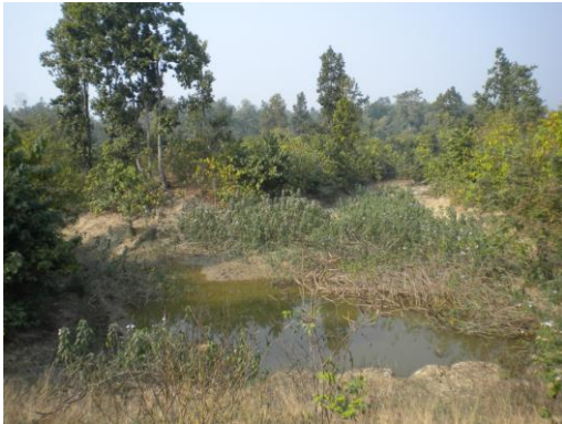
Runoff harvesting dam /Conservation storage
