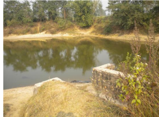
Runoff harvesting dam and conveyance
