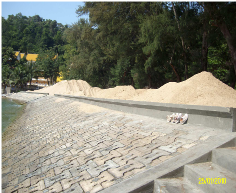
Figure 4-15 Seawall in Laem Sadet beach Source: Marine Department (2010)
