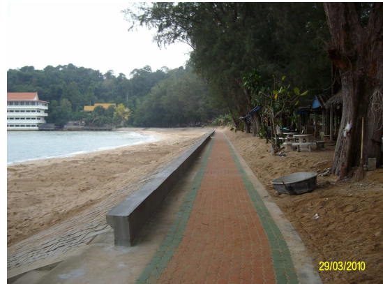
Figure 4-23 seawall of the building finished
