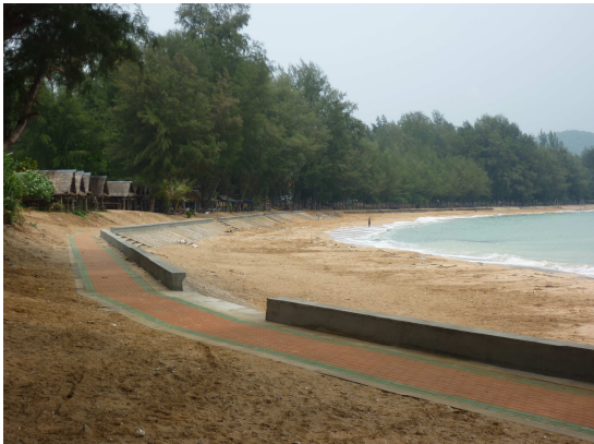
Figure 4-22 seawall of the building finished
