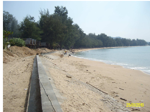
Figure 4-16 Seawall in Laem Sadet beach Source: Marine Department (2010)
