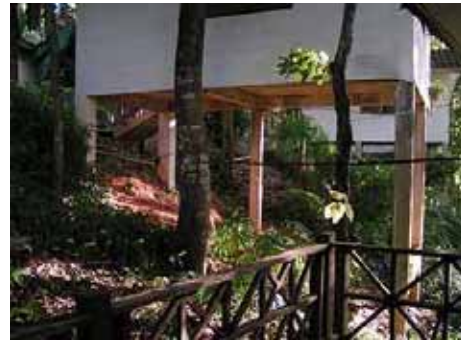
Figure40, 41: Typical Kuti/cottage at Vipassana accommodations (Level 5). Each Kuti sits on pilings for maximum ventilation and dryness.
