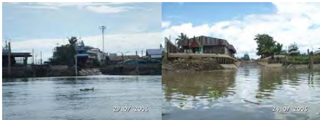
Figure 35 A few boats are berthed on certain sections of the Mae Klong River for repair or cleaning
