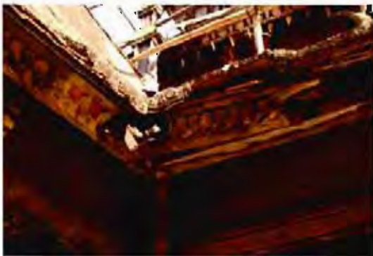
Figure 10: Eave and roof valley
