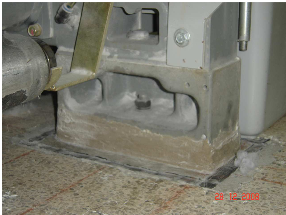
Figure 3-8 Installations the rubber valve plate at the machine base
