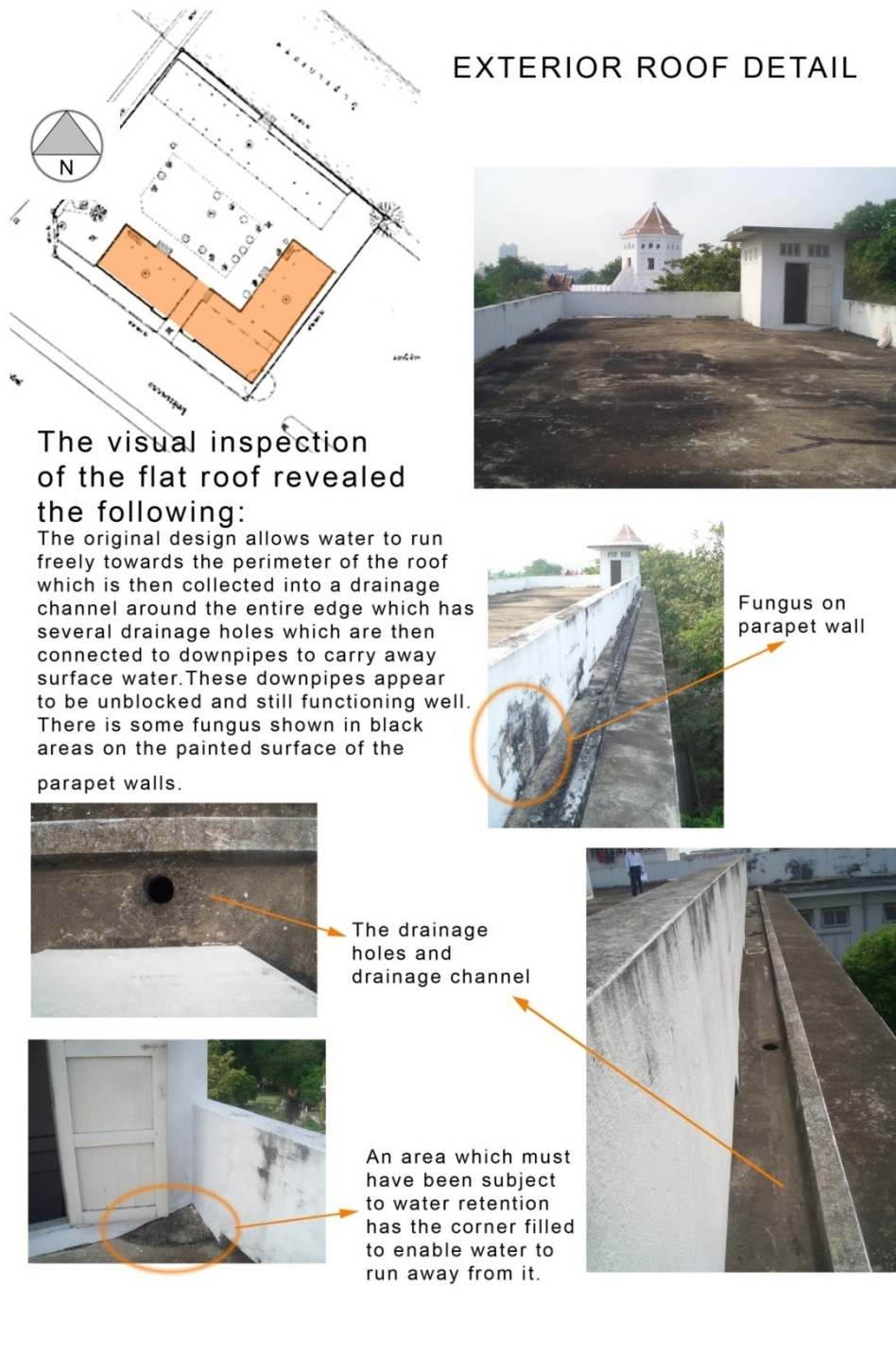
Figure 12 Kuru Sapha - Exterior roof details (author)
