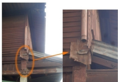
Flashing added which may need to be made more secure to prevent water penetration into the building
