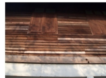
The timber siding and the concrete beam
