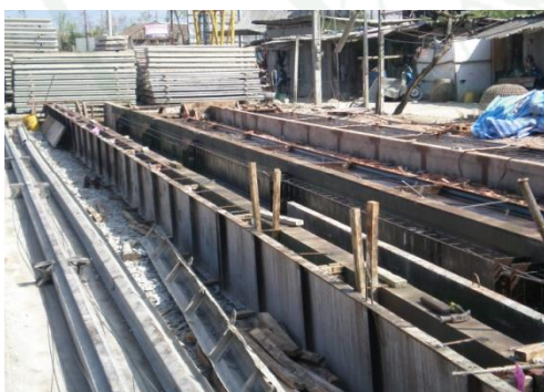
Appendix Figure 21 Rebar fixing and formwork
