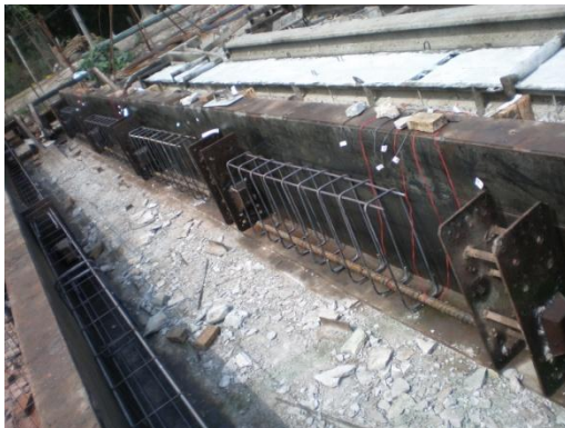
Appendix Figure B19 Rebar fixing and formwork
