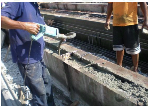
Appendix Figure B26 Concrete placing
