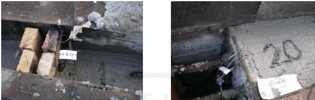
Appendix Figure B28 Concrete placing and identification
