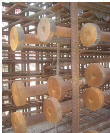
Figure 11 Headed bars in bridge structure
