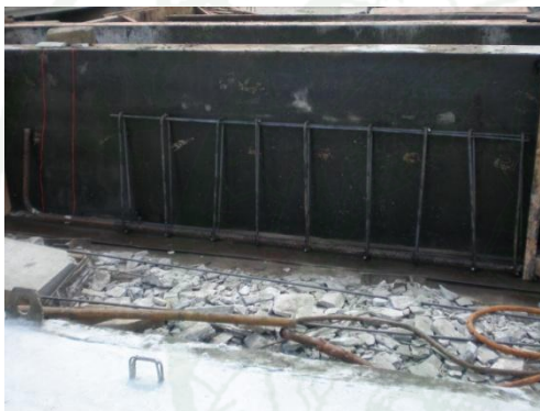
Appendix Figure B17 Rebar fixing
