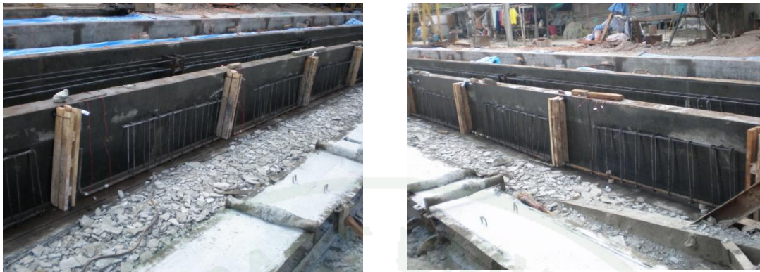
Appendix Figure B22 Rebar fixing and formwork
