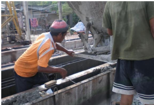
Appendix Figure B25 Concrete placing
