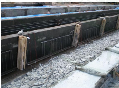
Appendix Figure B18 Rebar fixing
