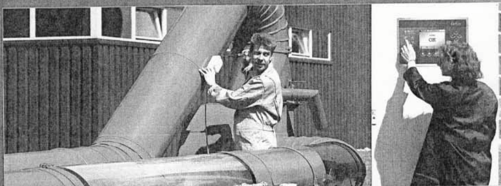
Experimental station - permanent development
