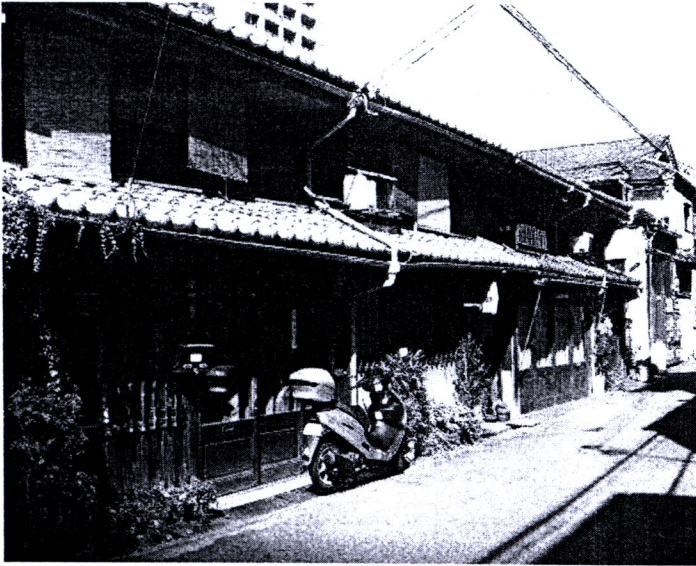
Figure 5.4: Conventional houses in the old alley, Osaka, 2010
